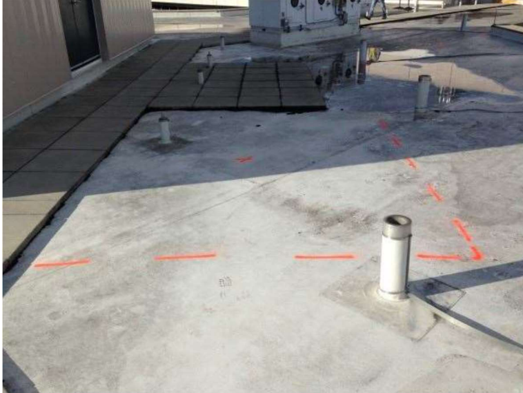
Picture showing wet area #1 on roof area A
